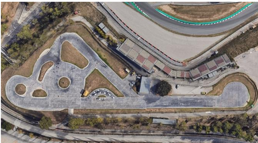
Figure 30 Aerial views of the Advanced Driving Centre in Montmeló
