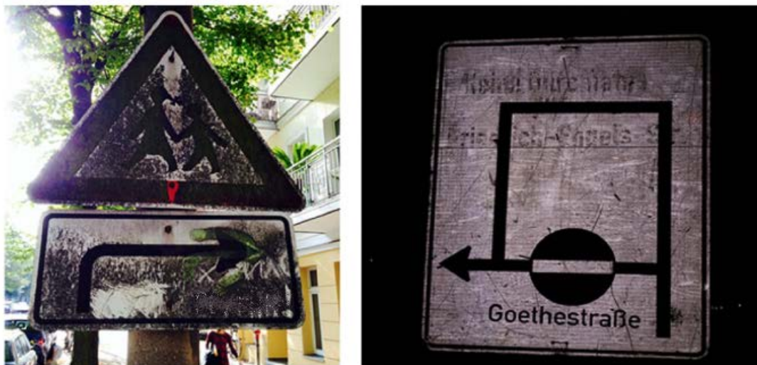
Figure 7-4: Examples of defective signs via Schilderüberwachungsverein [39]
